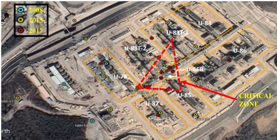
Figure 2. Critical zone of the parcel, considering explorations performed on 2008, 2015 and 2017.
