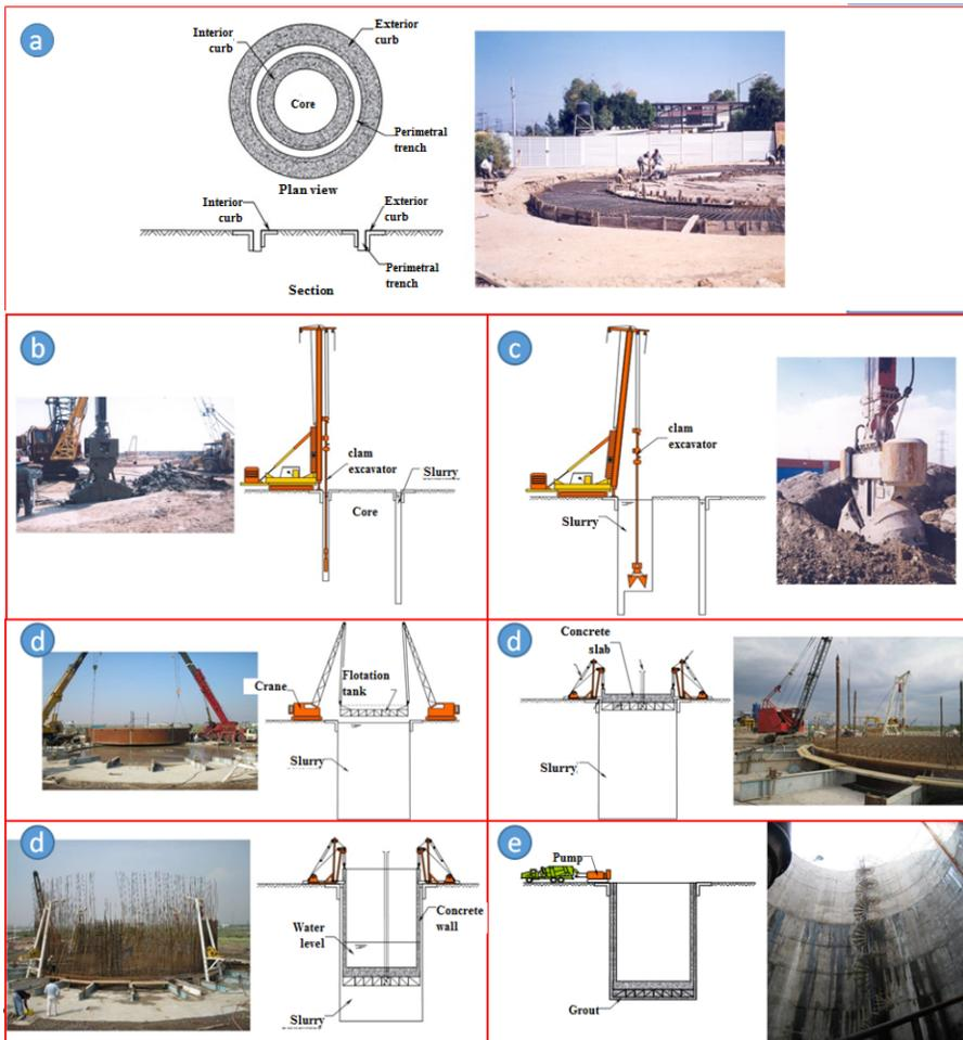
**Figure 3.** Construction stages of a tunnel shafts with “Flotation Method” (Modified from [1]).
