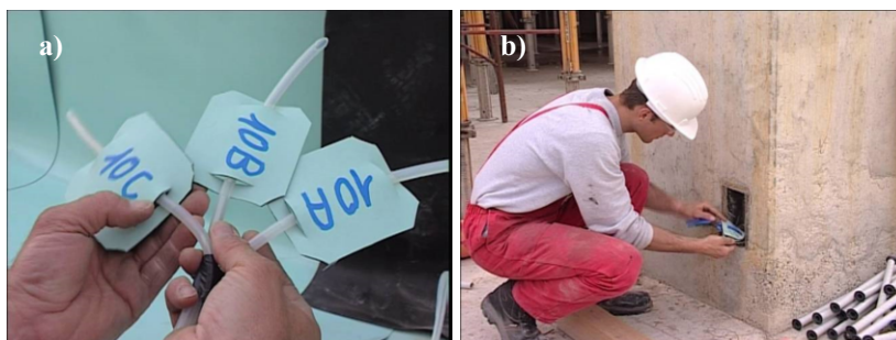
Figure 5. a) injection pipes numbered for each sector, b) positioning of the box in the structure.
