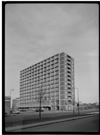
Figure 3. Osdorperhof nursing home in Amsterdam by architects J.W.H.C. Pot and J.F. Pot-Keegstra, 1962-1968. Stadsarchief Amsterdam, 5293.FO.
