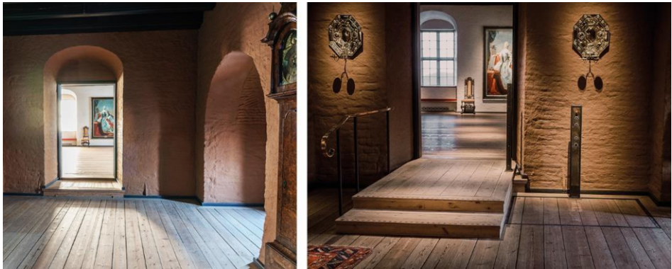
Figure 3. L.h.s: One of the halls before intervention. R.h.s.: A lifting platform is integrated in the floor. (Photo 1: Oslo Byggetreprenør AS; 2: A.M. Malkenes Mathiesen/The Norwegian Defense Estates Agency)
