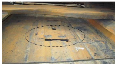
Figure 1. Impact damage of scraper conveyor [3] .
