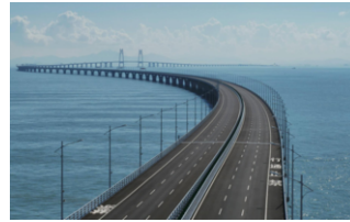
(b) Hong Kong-Zhuhai-Macao Bridge Deck Pavement
