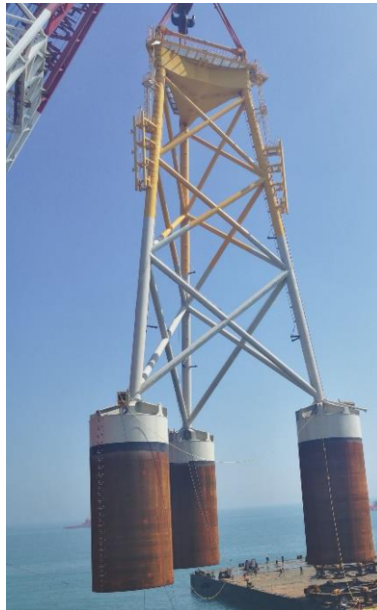
Figure 1. Suction pile jacket foundation.
