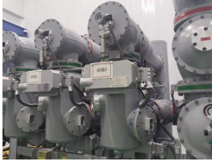
Fig. 7. GIS PD experimental platform.
