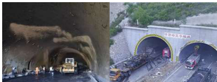
Figure 3. No. 5 Futuyu tunnel explosion accident.
