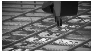
Figure 4. Tybot Developed by Advanced Construction Robotics.
