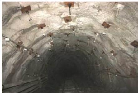
**Figure 13.** Repair effect of the field roadway
