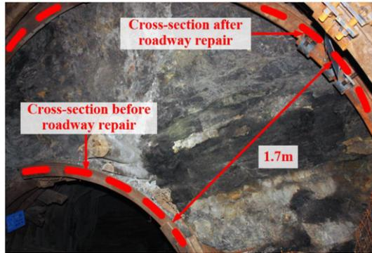
Figure 3. Cross-sections before and after roadway repair
