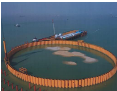
Figure 2. Island-building cofferdam closure of deep-sea anchorage. (Photograph: Shen-Zhong Link Management Center, China.)
