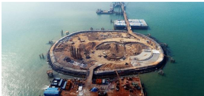
Figure 3. Island cofferdam with west anchor. (Photograph: Shen-Zhong Link Management Center, China.)
