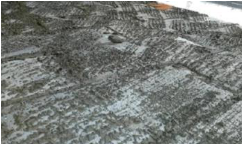
Figure 4. Grouting to finish the surface.
