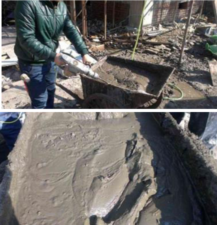
Figure 3. Stir to finish the paste.
