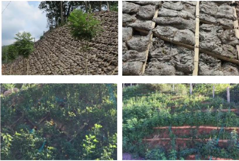
Figure 6. Utilization of waste materials used in slope protection of Xiaomo highway.
