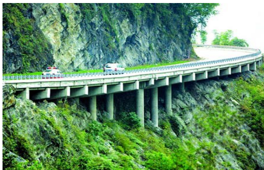
Figure 3. Half-roads and half-bridges adopted in the Shenlongjia highway of Hubei.
