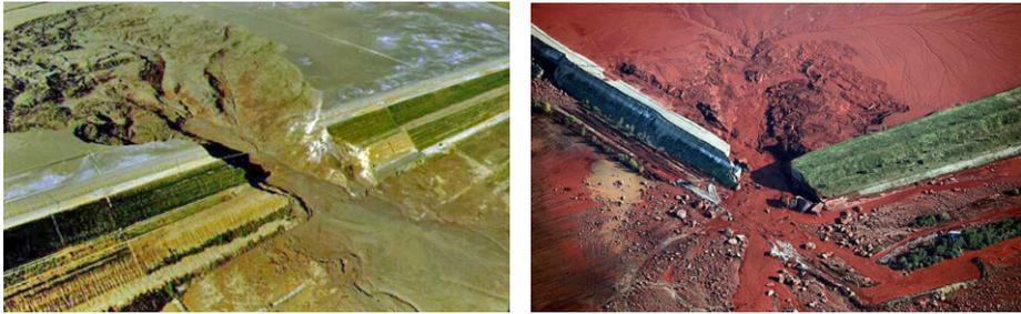
**Figure 6.** Flow liquefaction failures: a) Kolontar Tailings Dam failure in Hungary [24] and b) Harmony, Merriespruit, South Africa [25].
