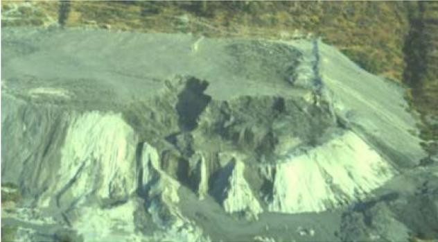
**Figure 1.** Seismic failure of Cerro Negro Tailings Dam [1].
