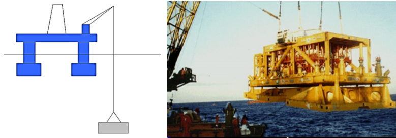
Figure 5.1: Lifting method
