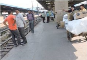
1. The volunteer C due to absence of any warning tactile strip is unable to identify the platform edge
