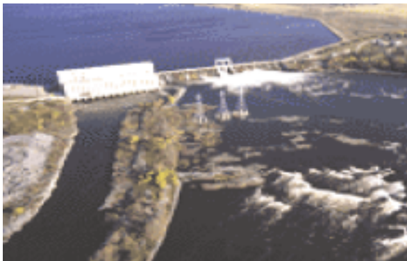
Figure 1: Powerhouse, forebay, and retaining dykes, Seven Sisters Generating Station
