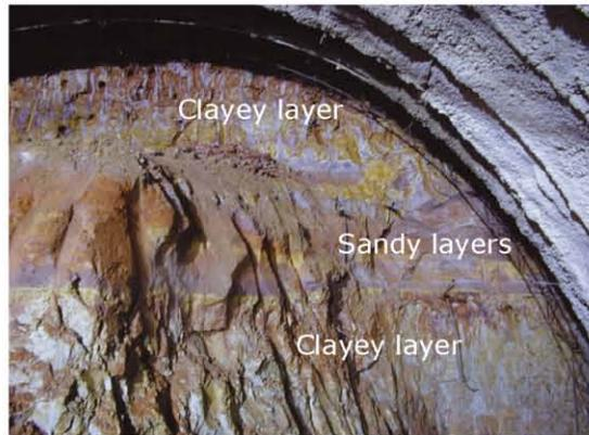
Fig. 10.4.2. Heterogeneous soils
