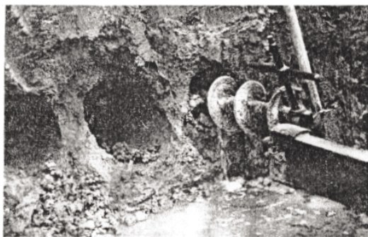
Figure 6. Changing of the foundation stability by drilling horizontal holes.
