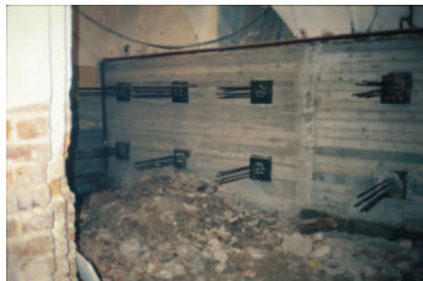
Photograph 3. Concrete beam h \times b = 2,0 \times 0,5 m 2 against the old cellar wall and pre-tensioned anchors.
