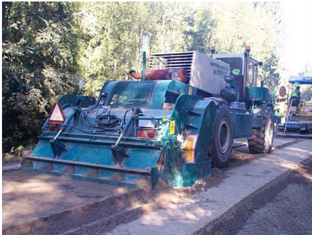
Figure 2: On-going stabilising process (Kukkia Circlet, Pilot 2002)
