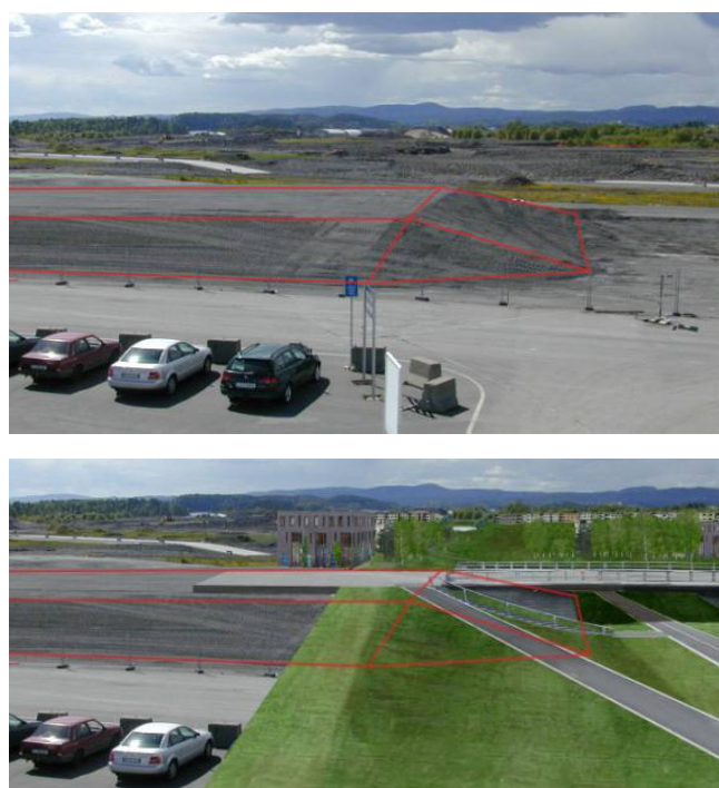
Figure 7 Use of PAH-contaminated soil in road construction at Fornebu, present situation (top) and future situation (bottom)
