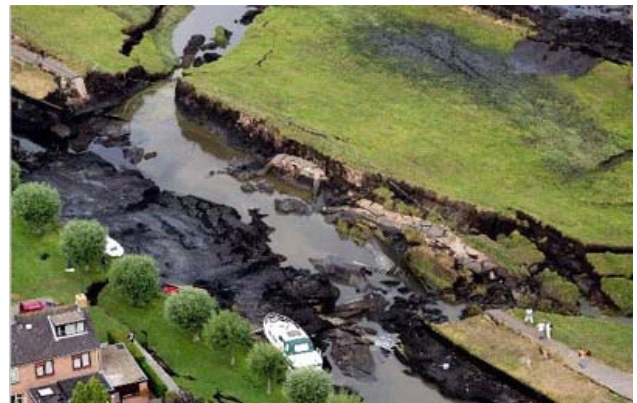
Figure 4. Canal embankment collapse at Wilnis, 26 August 2003.
