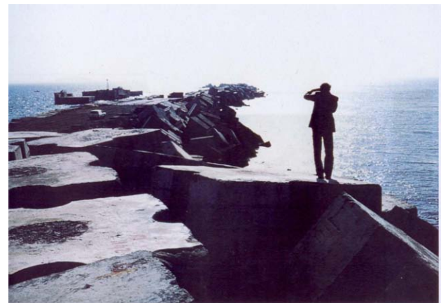
Figure 17. Breakwater at Sines, the world's largest, after failure in 1982
