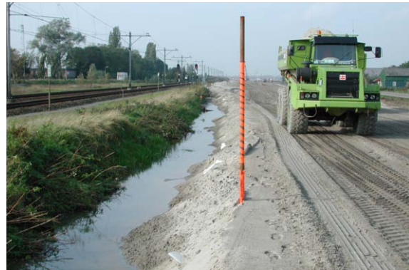
Figure 41. The new Betuwe line runs close to existing infrastructure; by applying a monitoring concept to the largest risk factor: the subsidence, a new type of PPP contract could be established, leading to significant cost reduction and an excellent project result.
