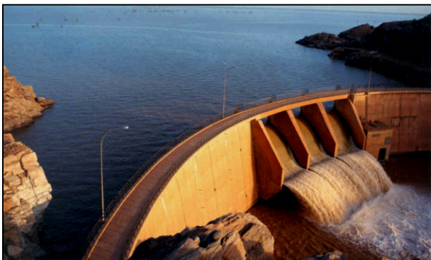
Figure 1. Foug Gleita arch dam
