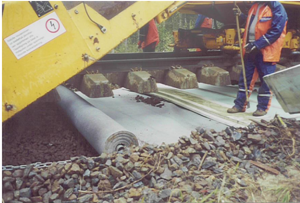
Figure 2. Installation of frost insulation boards under the ballast layer during ballast cleaning.
