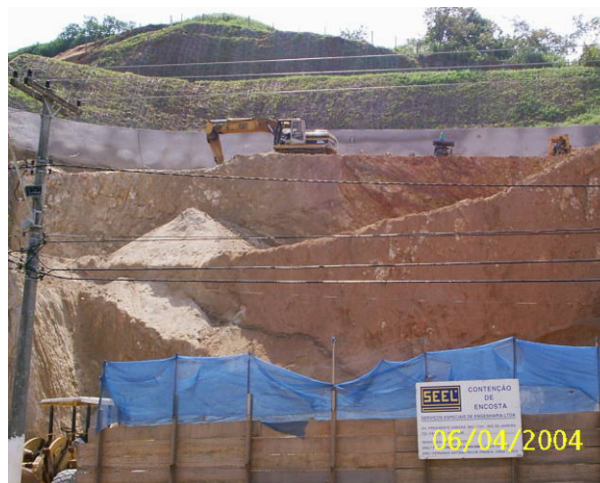
Figure 6 – First stages of nailed excavation.
