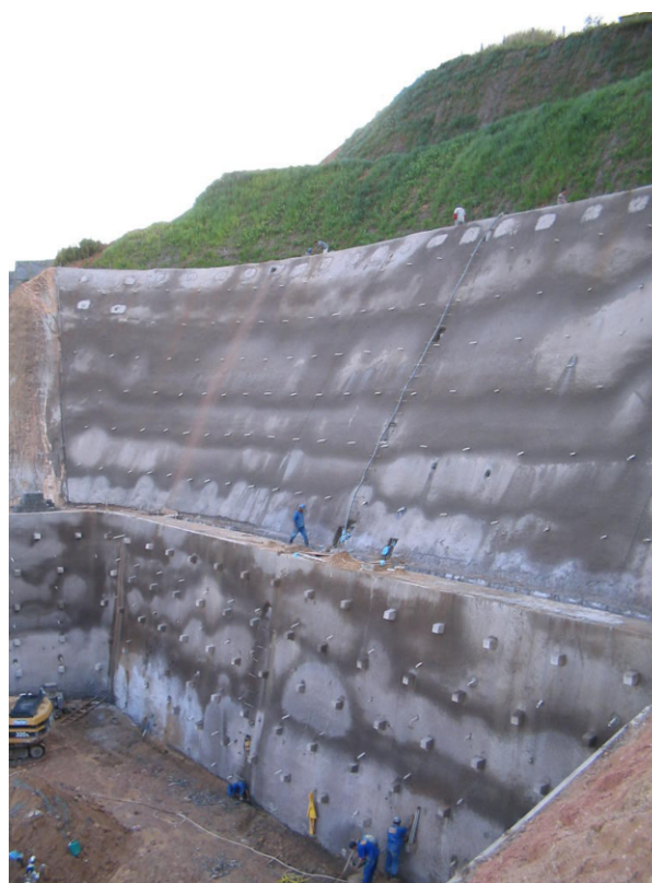
Figure 7 – Last stages of 40m high nailed excavation.
