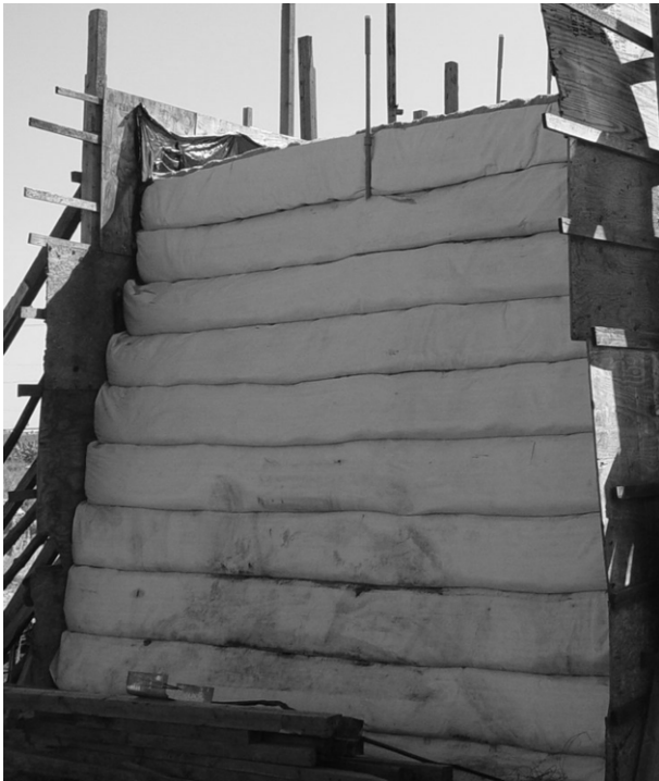
Figure 1 – Geotextile reinforced soil retaining wall
