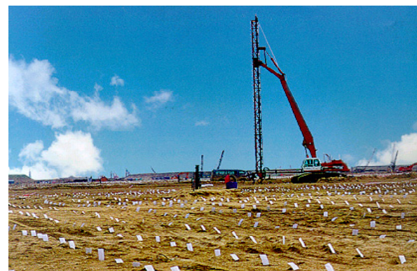
Fig. 3 Installation of plastic board drain
