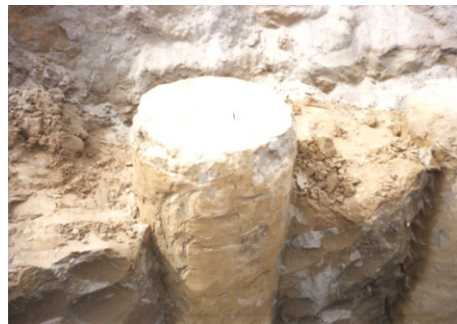
Figure 6. DMM column head before loading test
