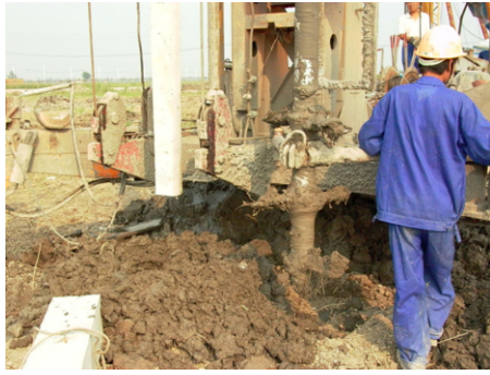
Figure 7. Mini pile driving after DMM column installation
