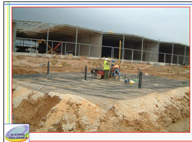
Figure 13. Static railway full scale load test: LTP under construction.
