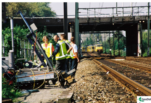
Figure 3: Execution of an inclined CPT.
