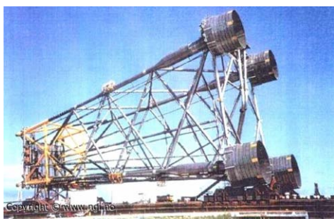
Figure 4.9 Draupner E jacket with steel bucket foundations (© NGI)
