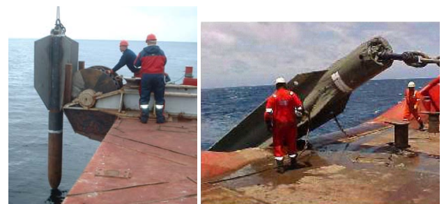
Figure 6.16 Dynamically penetrating anchors (a) field trial (O'Loughlin et al., 2004); (b) installation of torpedo anchor (Medeiros, 2002)
