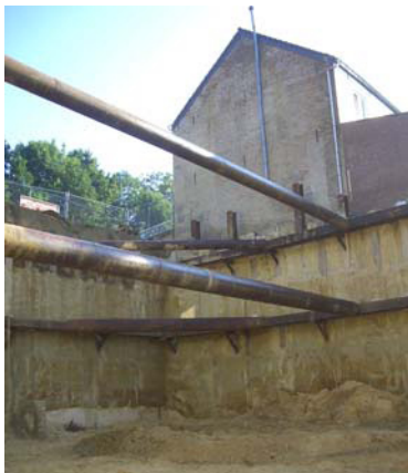
Fig 9: CSM wall (Holland) after excavation
