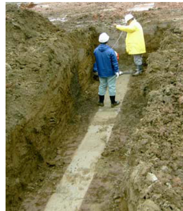
Fig 8: Exposed top of CSM wall in silty clay
