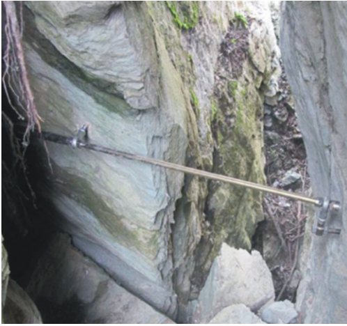
Figure 3. Photo of one extensometer within the crack in the Head Area .
