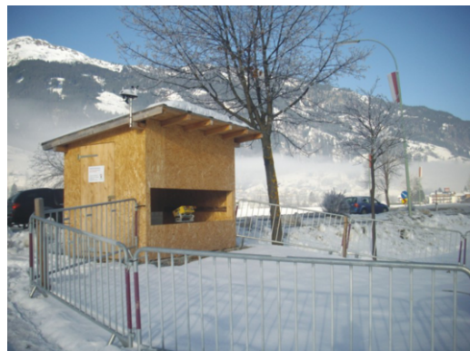
Figure 2. Photo of installed equipment.
