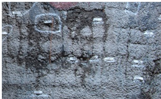
Figure 6. Location of reinforcement bars visible in Panel 2
