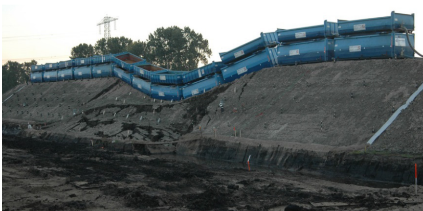
Figure 11: Full-scale test embankment failure at the IJdijk facility in the Netherlands. For more information refer to Zwanenburg et al. (2012). Source: Deltares.
