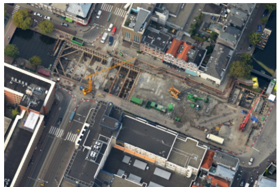
Figure 5. Excavation in 2 compartments
