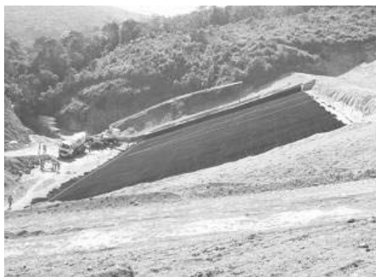
Figure 9. Concrete pumping system placed.
