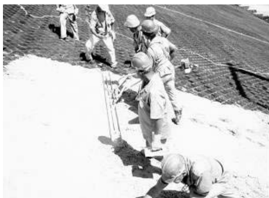
Figure 10. Vibratory rule being use.
