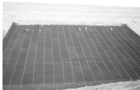
Figure 7. Geocells expansion/ Geotextile placed.
