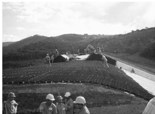
Figure 12. Detail of the geocells flexibility.
