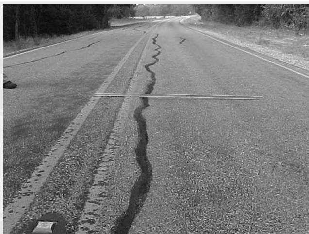
Figure 1. Typical longitudinal crack developed on pavements over expansive clays.
