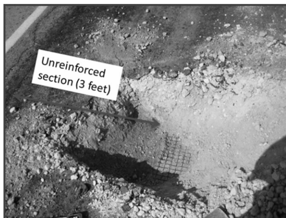
Figure 5. View of edge of geogrid reinforcement, directly underneath longitudinal crack.
