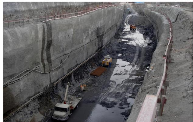
Figure 3.4: A general view of the supported shaft walls on completion of the excavation (Taheri *et al.*, 2009).
