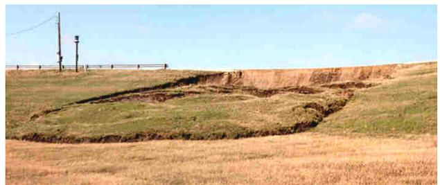
Figure 3.8: A typical surficial failure at Joe Pool Dam (Puppala *et al.*, 2009).
