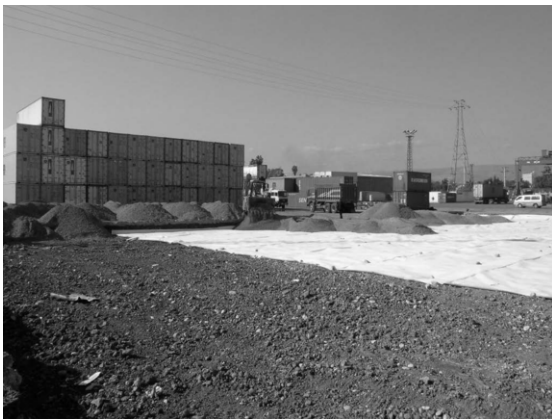
Figure 15. Installation of composite base course reinforcement (Source: Fig. 7, Heerten et al.)
