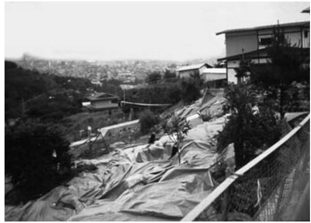
Figure 4.28: Collapsed houses due to slope failure at Midorigaoka in Sendai City during the 1978 Miyagiken-oki earthquake
