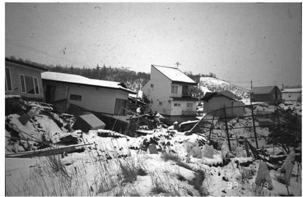
Figure 4.35: Deformed bank and damaged houses at Kayanuma during the 1993 Kushiro-oki earthquake
