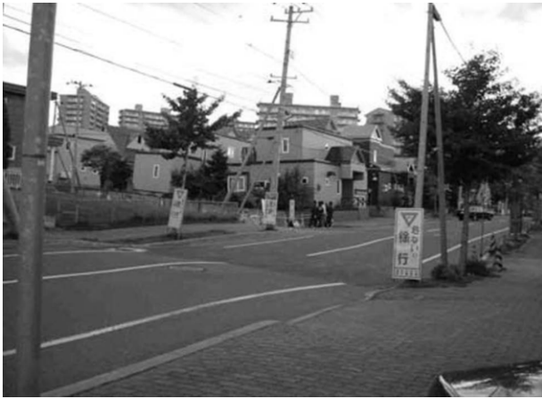
Figure 4.26: Settled houses due to liquefaction during the 2003 Tokachi-oki earthquake at Utsukushigaoka district
