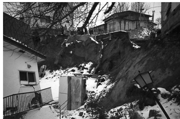
Figure 4.31: Failed slope and damaged houses at Midorigakoka in Kushiro City during the 1993 Kushiro-oki earthquake
