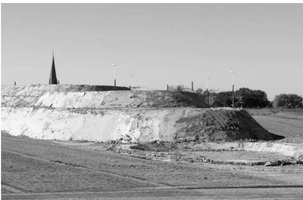
Figure 1. Landscaping with stabilized soil.
