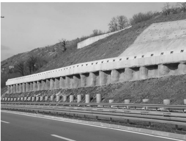
Figure 6. Photo of pile-wall construction in the toe of the landslide.
