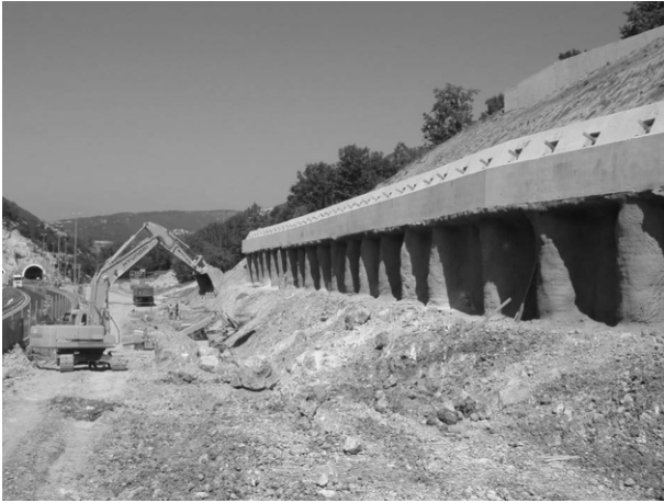
Figure 5. Photo of pile-wall during construction.
