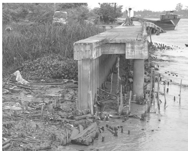
Figure 1. Road widening and riverbank protection using corrugated concrete sheet pile and concrete spun piles.
