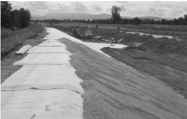
Figure 2. Rehabilitation of dike slope along the Kinzig River (2001): covering of the GCL Bentofix with gravel as an "animal deterring" cover layer (right)
