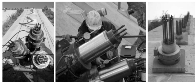
Fig. 9. Stressing the Anchors
