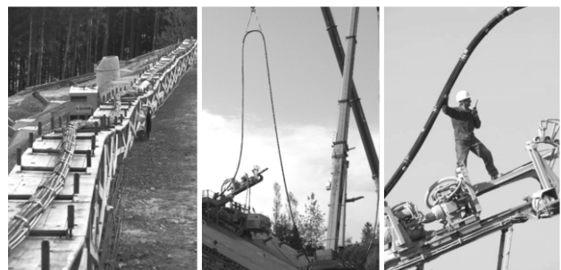
Fig.10. Assembly and installation of anchors
