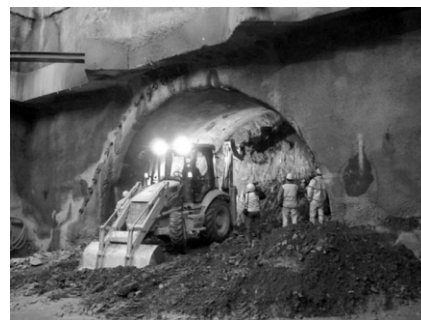
Fig. 8 - Test tunnel under excavation
