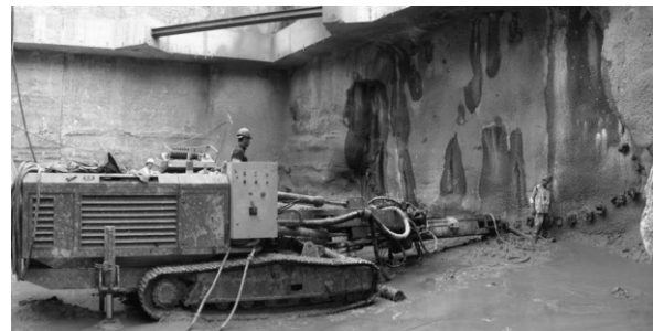
Fig. 7 - Positioner carrying out HJG at the invert
